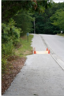
Final piece of Village Drive Sidewalk nearly complete
