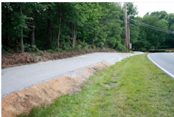
New Kingsboro Sidewalk Trail-bed Waiting for Final Blacktop Paving
